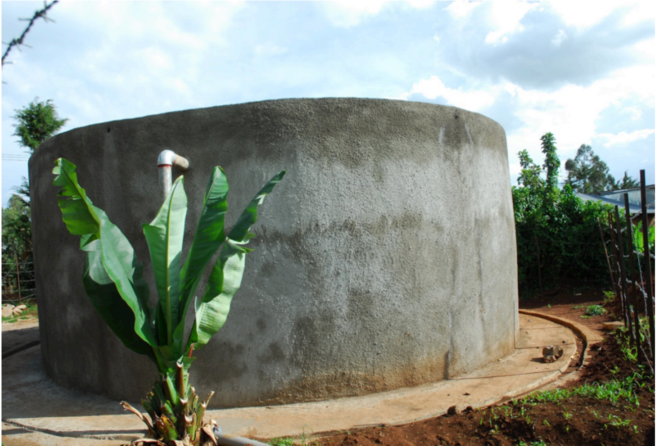
Concrete Water Reservoir constructed for community by ActionAid
